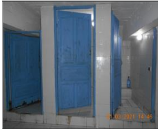
Photo of the sanitary facilities sanitary area.JPG
